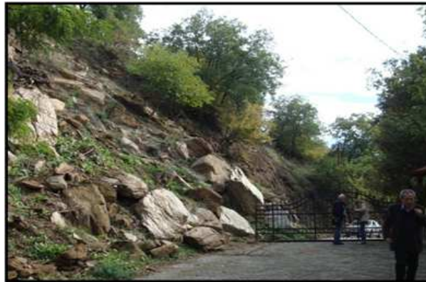
Image 1: The Foot of the Landslide at the Entrance of the Camp. The Material of the Landslide Consists of Big Volumes of Mica Schist Combined with Soil Weathering Material
