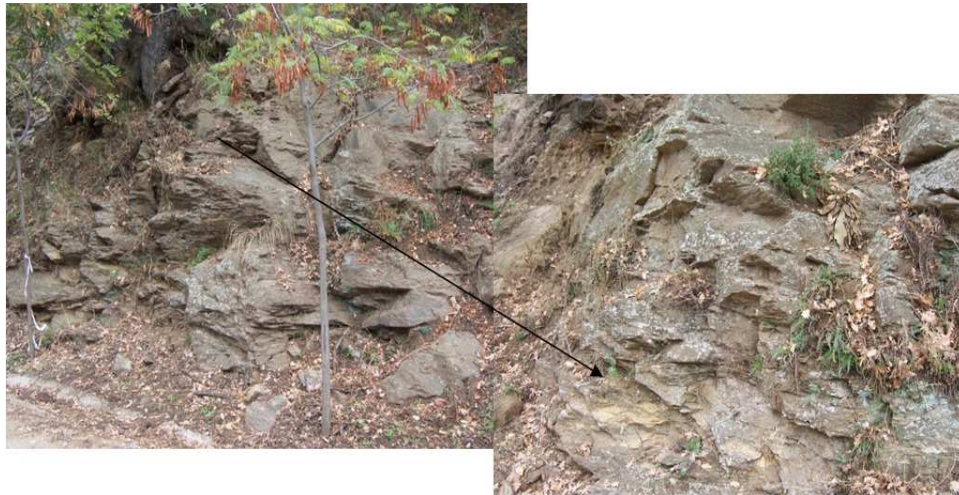
Image 3: The Mica Schists Right from the Eastern Boundary of the Landslide (in Detail the Discontinuities)
